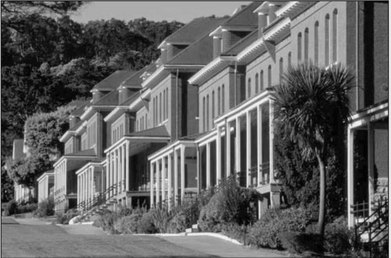
Colonial Revival style enlisted men's barracks (1895) lining Montgomery Street edge of Presidio's Main Parade Ground, greeted visitors to Presido Trust's first public open house.
