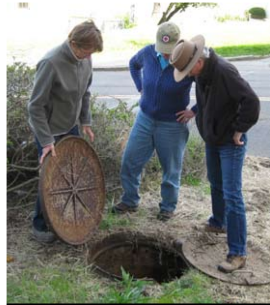
Field crew members Garrett observing part of the defense communication system
