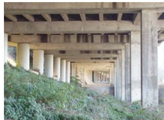
Columns visible from Bank Street beneath Doyle Drive
