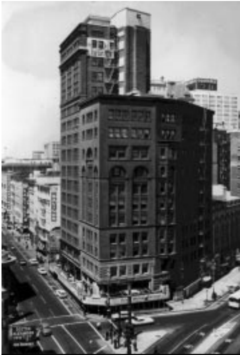
Photo on left shows Burnham design of Chronicle Building with Polk-designed tower addition and two additional floors to Market Street structure. Middle photo shows removal of cornices and other decorative details. Modernized building on right.
