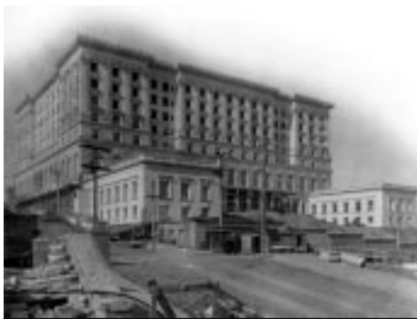
Hotel undergoing reconstruction, February 7, 1907
