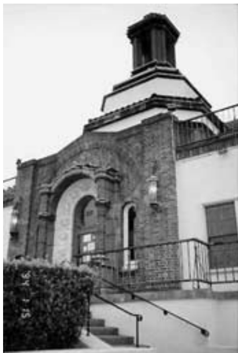
Ortega Street entry to the San Francisco Infant Shelter (Mullgardt: 1927)
