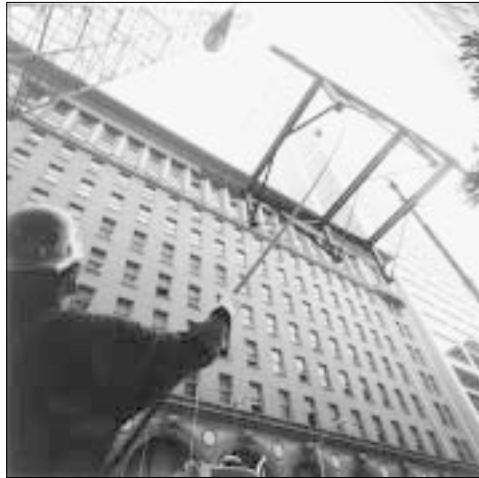
Hoisting platform (left) for one of two roof-mounted cranes, shown in place on right lowering drill rig into lightwell for installation of new piles in recently completed seismic retrofit of the Southern Pacific Building.
