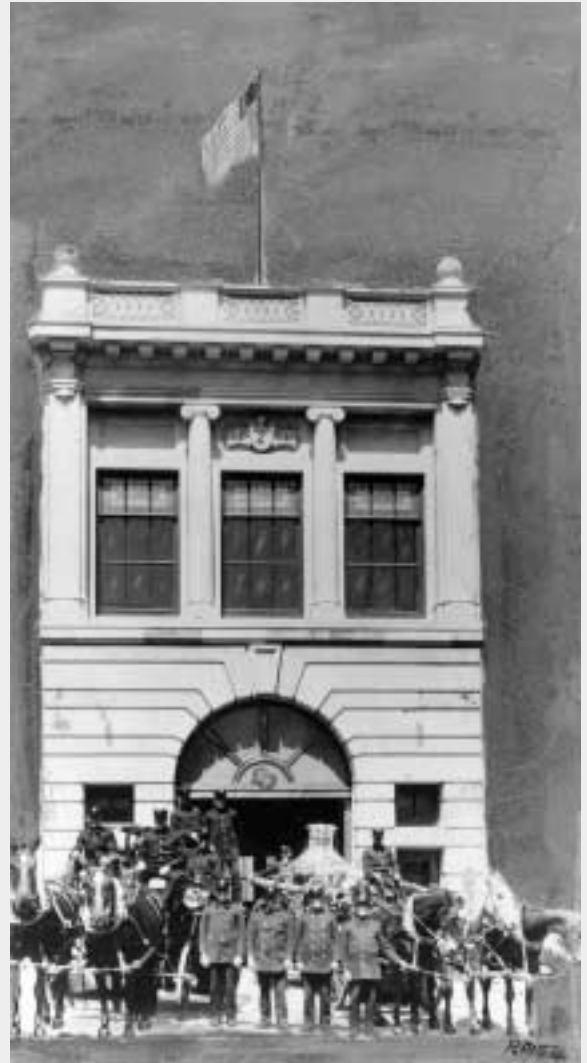
460 Bush Street, Engine Company No. 2 (c. 1910)
