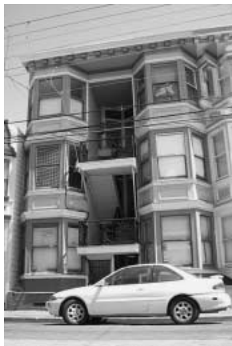
Typical "Romeo Flat" on Woodward Street. Photo: Planning Department
